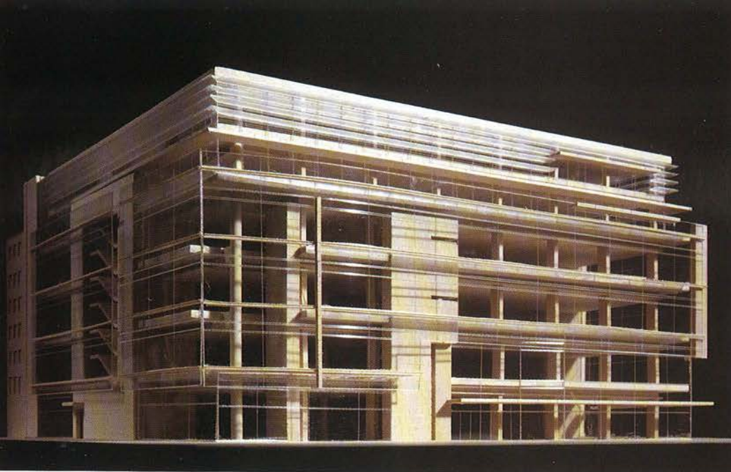
The Peek & Cloppenburg Department Store, in Mannheim, Germany (above), to open in 2004, features a three-story-high glass enclosure cantilevered from the main structure.
