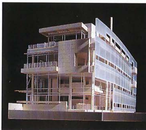
The Rickmers Reederei Headquarters, in Hamburg, Germany (right), has just been completed. Notable is an elegantly glazed screenlike wall.
